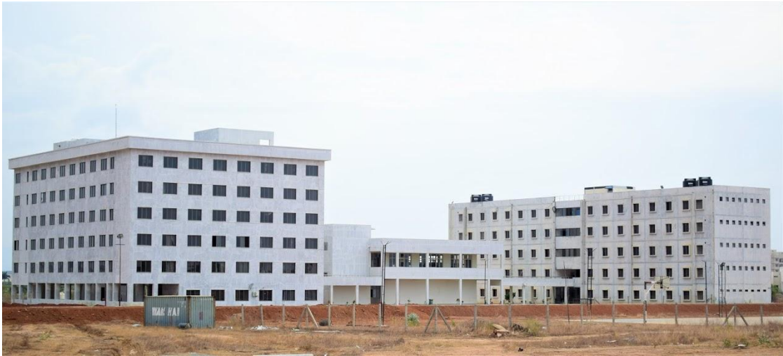
Hostels and Dining Hall Facility
